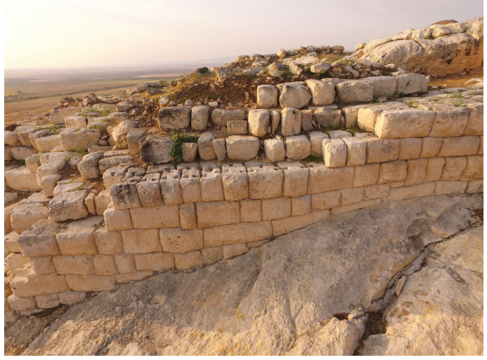
Figure 8. The highest part of the northern fortification wall: the rock-cut base, rustic elaborations of quadras, the facets and 'swallow-tail' connections.
