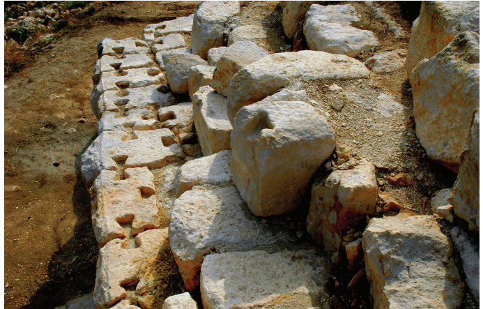
Figure 9. The horizontal polished surfaces of the quadros, rustic elaboration of outer faces, the facets and 'swallow-tail' connections: northern fortification wall.
