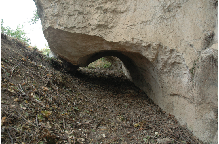
Figure 39. One of the tunnel parts of the canal.
