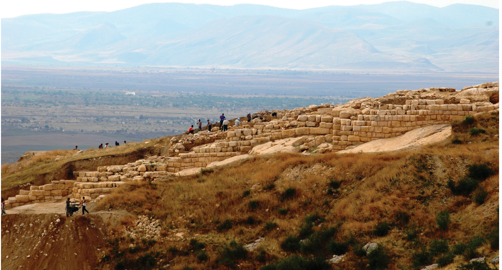
Figure 7. The upper part of the northern fortification wall, 2009.
